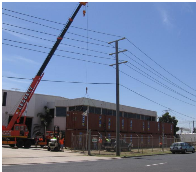
Figure 6 Shipping Containers Being Placed to Control LFN
